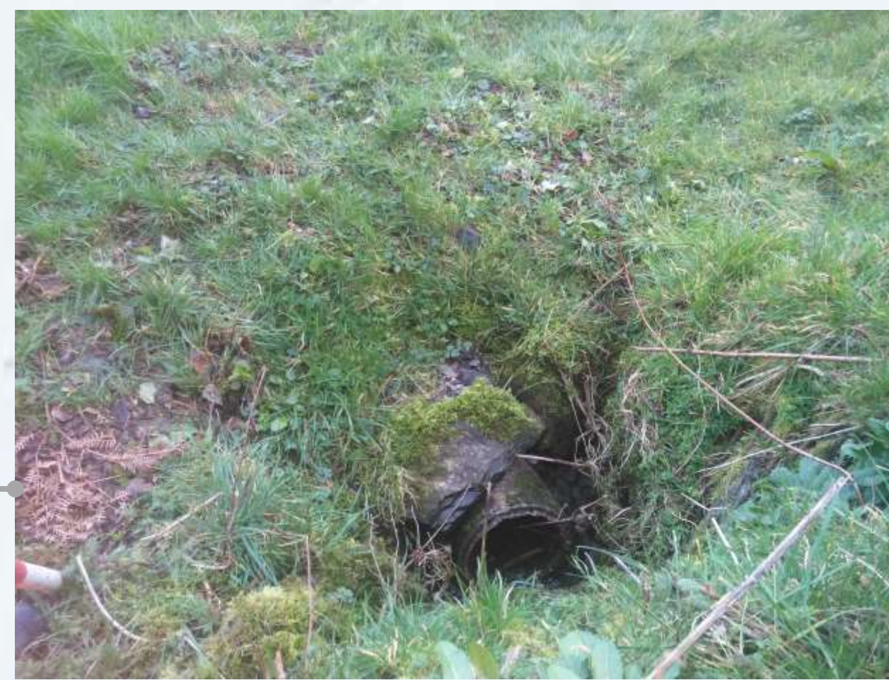
Upstream end of existing culvert
