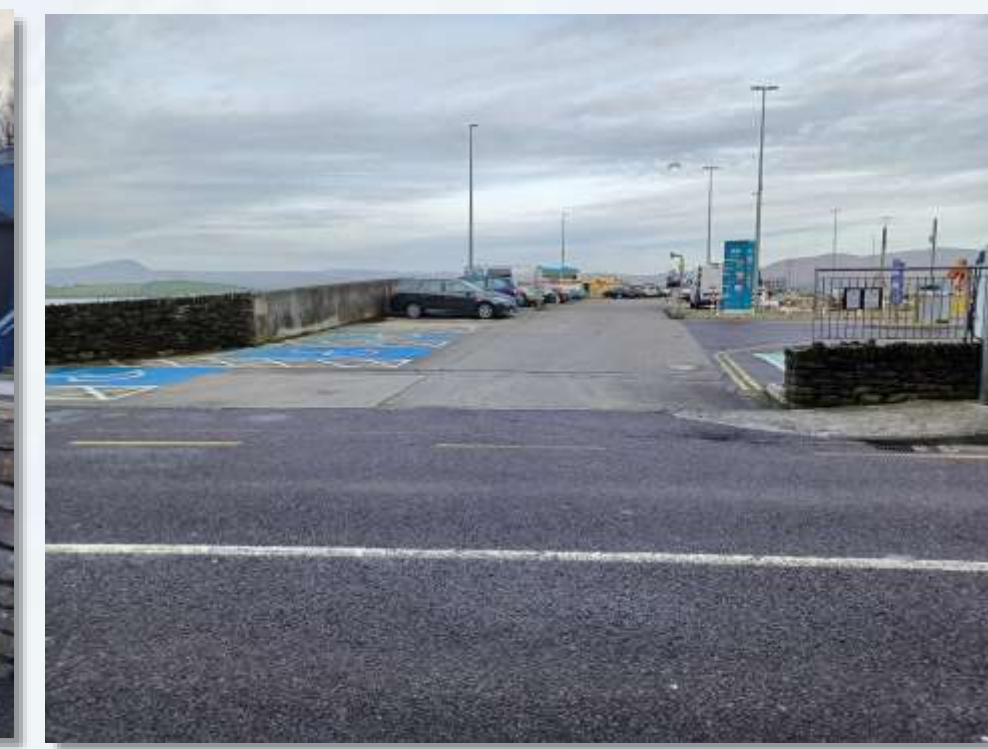
Entrance to Bantry Harbour Marina
